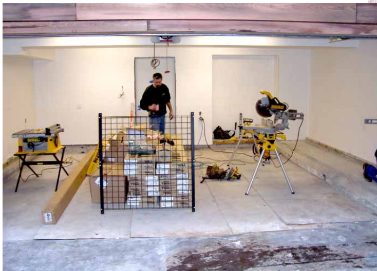
(left) Finished garage walls before garage organization.
